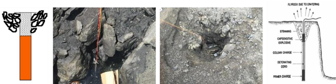
Fig. 1 Large benches and top priming causes flyrock [20]
