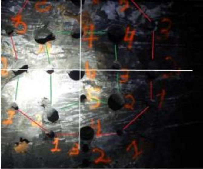
Figure 5: Execution of slot drilling with DL 421 at a lateral angle of 45°.
